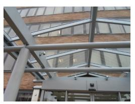
Working closely with the Leading London interior fit out company Cambs Glass bespoke division was contracted to carry out the removal of an existing barrel vaulted polycarbonate canopy with a modern dual pitched glass version to both modernise the office block entrance and to improve the functionality of the space bellow.
